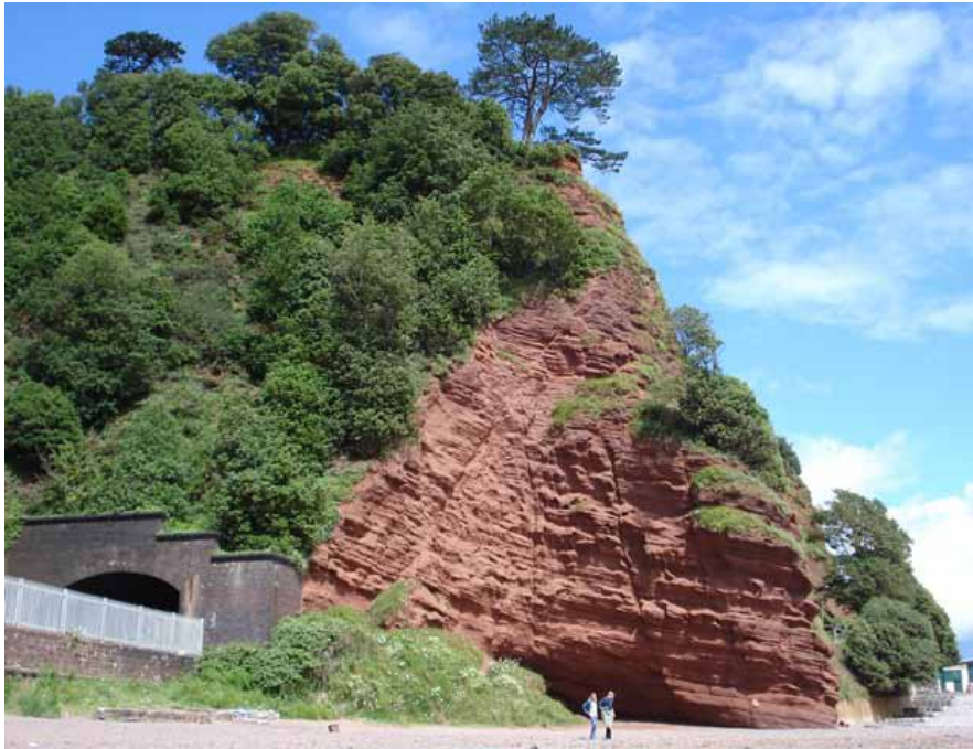
Easily erodible sandstones by the entrance to Kennaway Tunnel Jenny Lunn © RGS-IBG Discovering Britain
