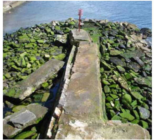
A concrete breakwater broken by the waves Jenny Lunn © RGS-IBG Discovering Britain
