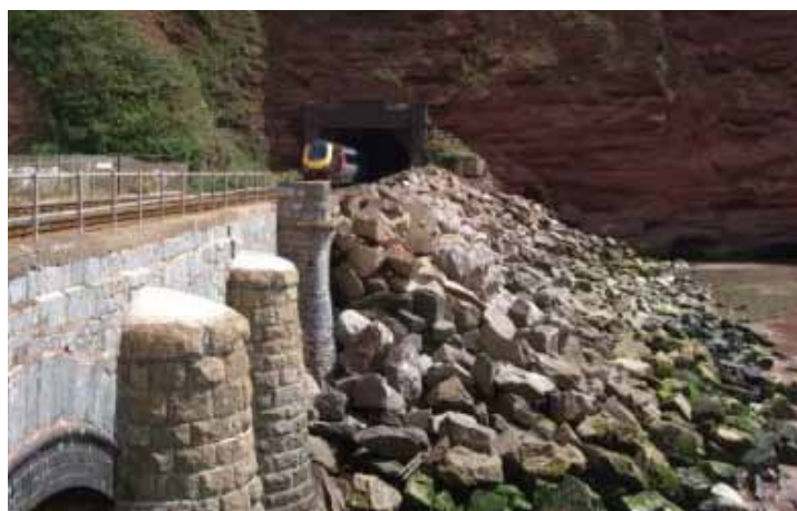
Rock armour near Parson's Tunnel Pat Wilson © RGS-IBG Discovering Britain
