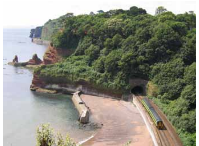
Coryton Cove and entrance to Coryton Tunnel © Stephen Craven, Geograph (CCL)
