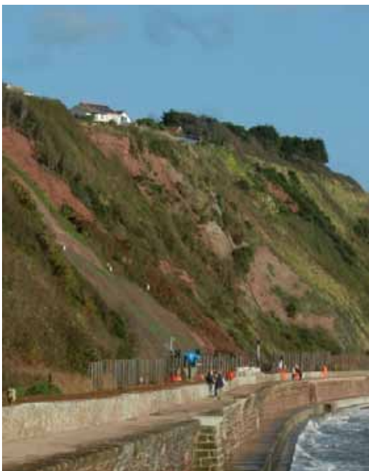
Work on some of the landslips that followed the 2014 storms - notice the house near the cliff edge Pat Wilson © RGS-IBG Discovering Britain
