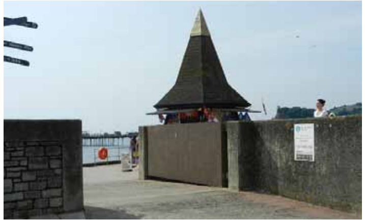
The seawall gate that protects Teignmouth town Pat Wilson © RGS-IBG Discovering Britain
