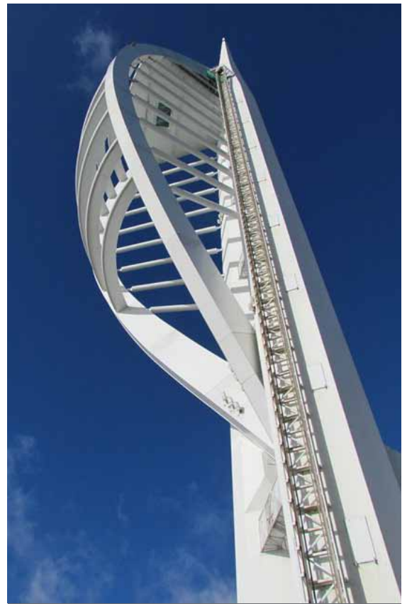
The Spinnaker Tower, the 'landmark building' of regenerated Portsmouth Rory Walsh © RGS-IBG Discovering Britain
