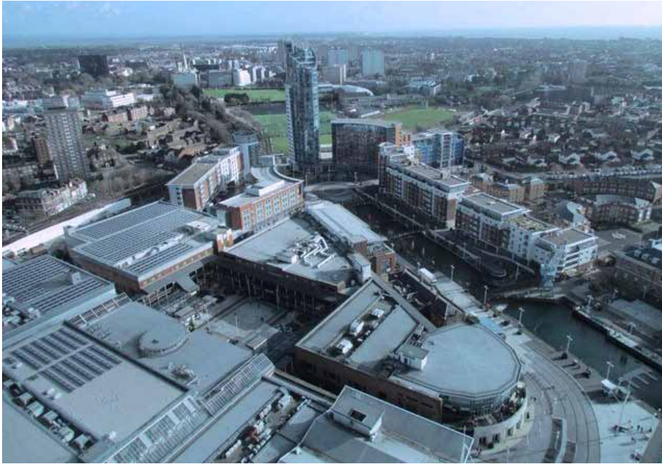
Gunwharf Quays as seen from the Spinnaker Tower indicates how large the dockyard used to be Rory Walsh © RGS-IBG Discovering Britain
