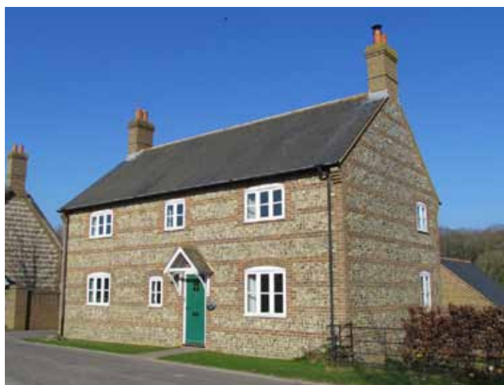
The two new flint cottages Rory Walsh © RGS-IBG Discovering Britain
