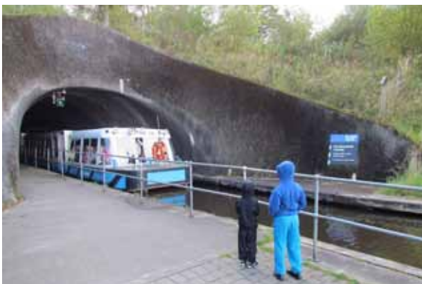
Roughcastle Tunnel © Rory Walsh
