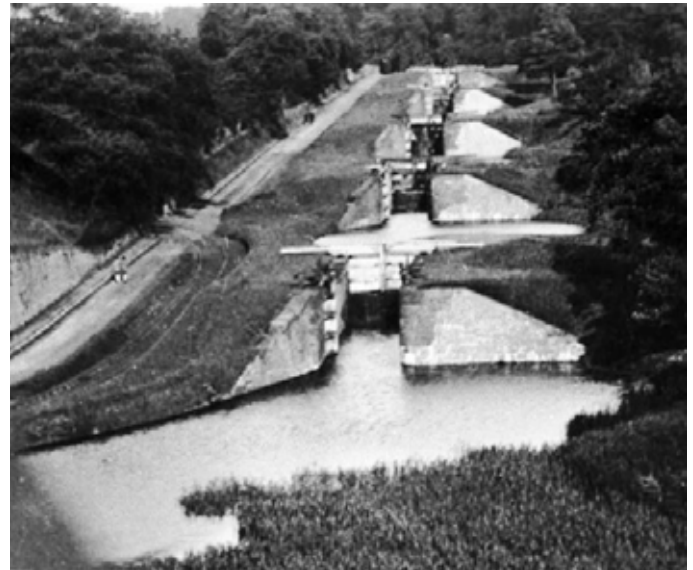
Junction Locks (c.1930) joining the Union and the Forth and Clyde canals Reproduced courtesy of Falkirk Archives
