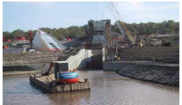
The Falkirk Wheel under construction © Sarah Charlesworth, Geograph (CCL)
