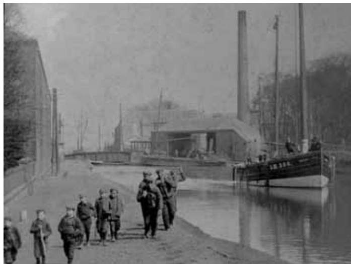
Forth and Clyde Canal at Camelon, Falkirk with sea-going boat (c.1910) Reproduced courtesy of Falkirk Archives
